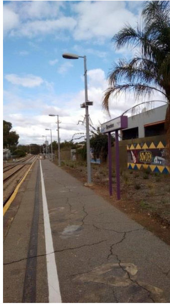
Photo 2. Cracked pavement
