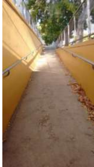
Photo 3. Underpass Street & platform (upwards)
