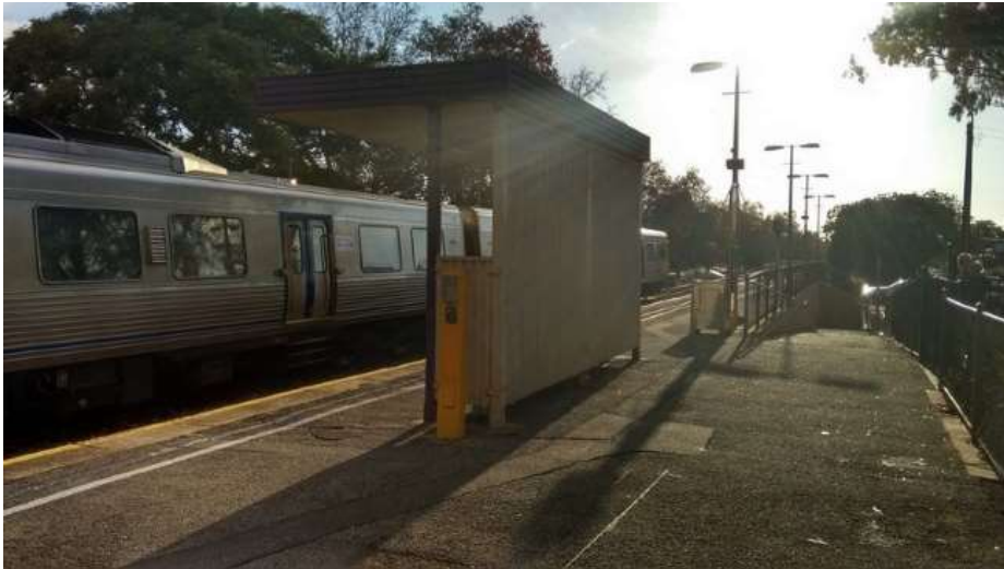
Photo 6. For the space available on the platforms the shelters are small and inadequate as well as downright ugly.
