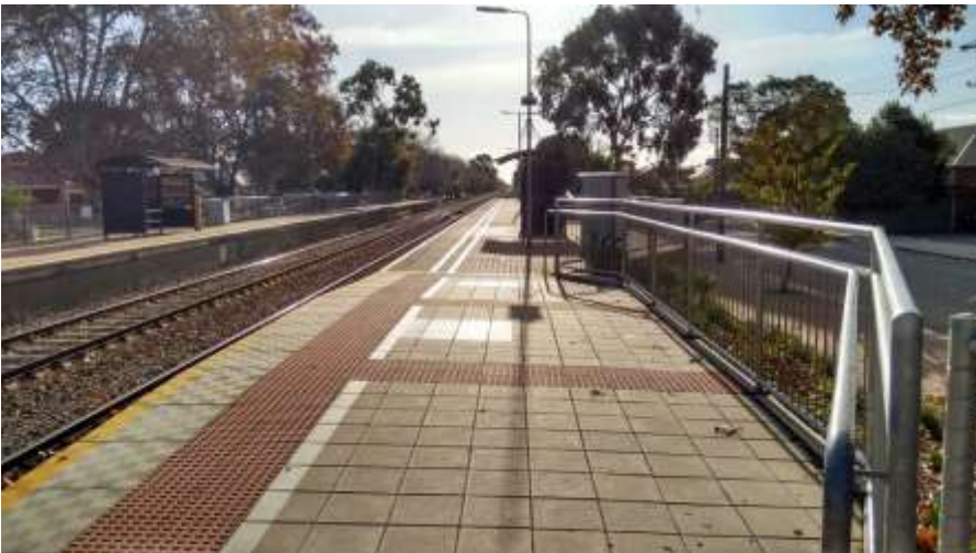
Photo 3. Wheelchair ramp –No shelter where it is most convenient for the disabled to wait.
