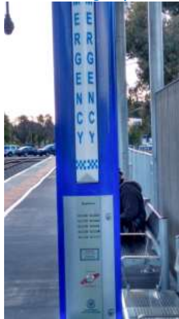
Photo 5. Emergency call button and intercom
