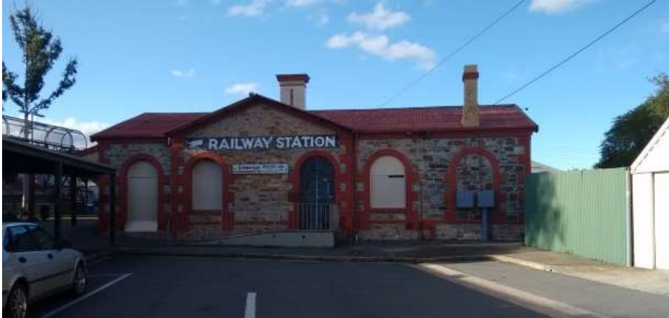
Photo 1. Grand approach with the the old station building. The current tenant is a barber shop
