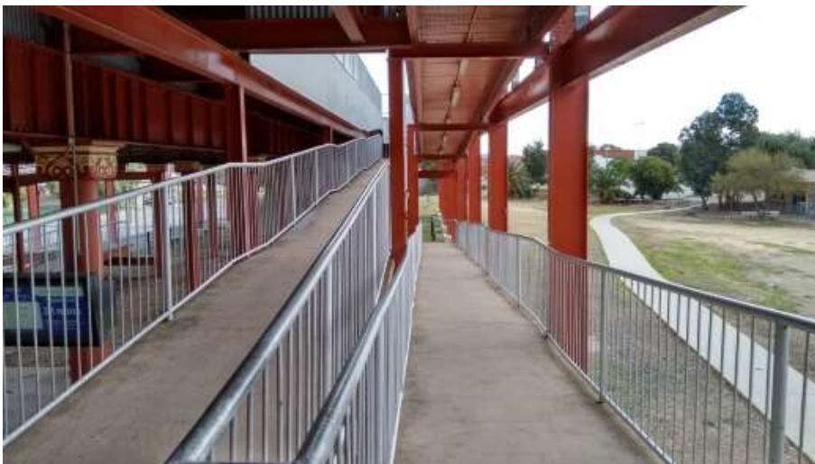
Photo 6. Long, long three tiered ramp to get up to the platform level. NO elevator in sight.
