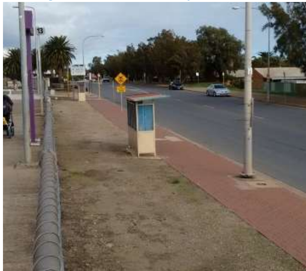
Photo 7. A lonely and substandard bus shelter next to the station. No integration with the railway station at all.
