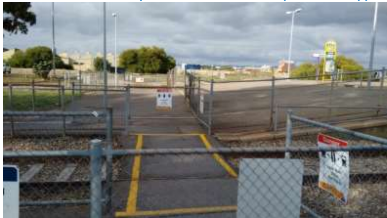
Photo 11. Access to all platforms from this one pedestrian approach (facing eastwards)
