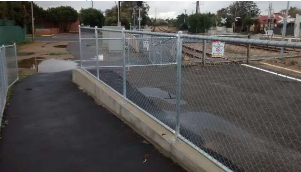
Photo 11. North East approach
