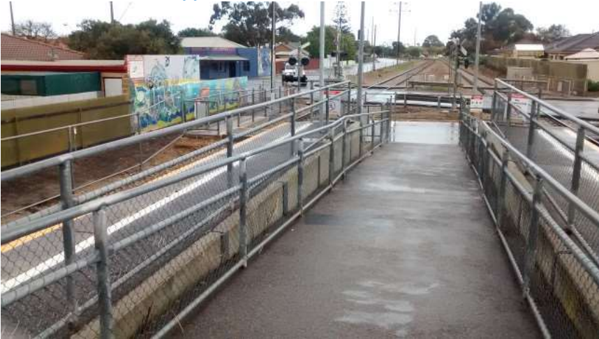
Photo 8. South East approach
