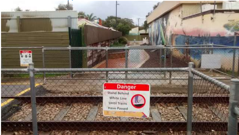
Photo 4. North East approach
