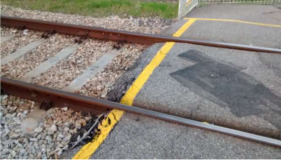
Photo 9. Broken asphalt
