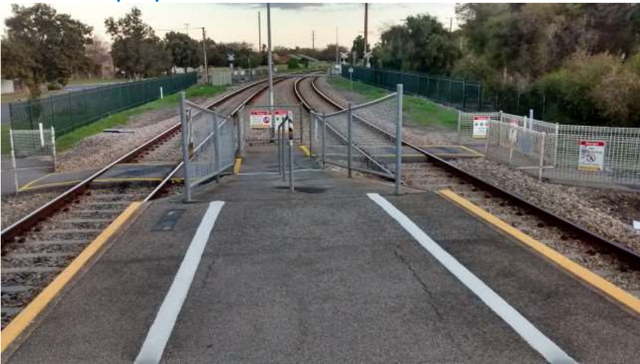
Photo 7. Ramp to platform
