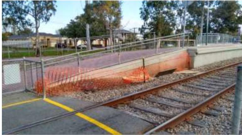
**Photo 12. Cracked pavement on platform. Wheelchair ramp NOT under a shelter.**
