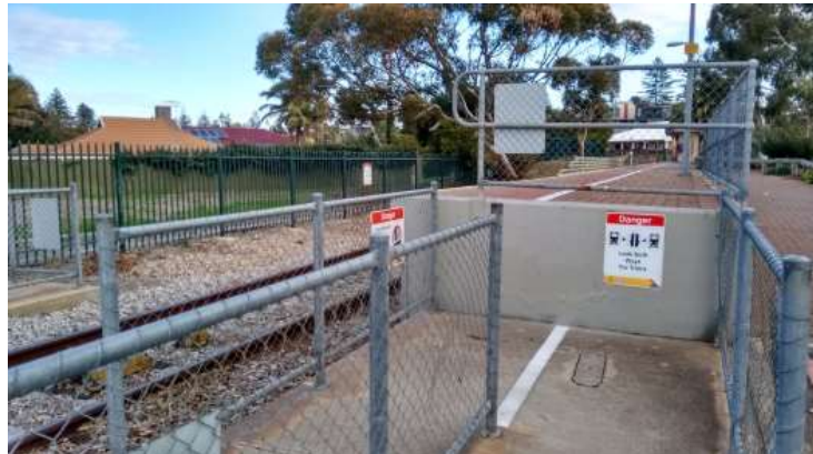
Pedestrian crossing towards the houses on the southern side of the line. This crossing is large enough and wide enough for wheelchairs and motorised scooters to move around in.
