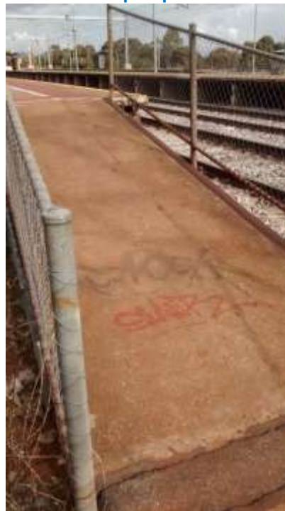
Photo 8. Ramp to platform 1
