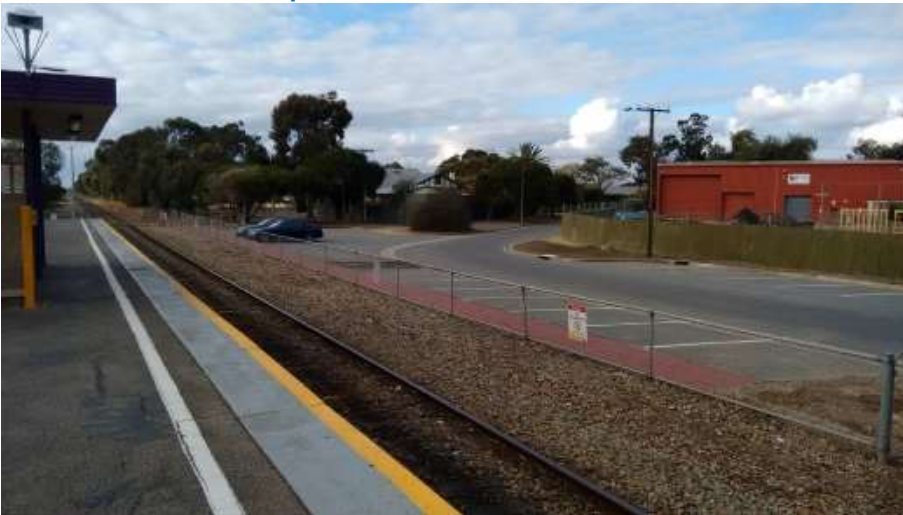
Photo 7. South East car park
