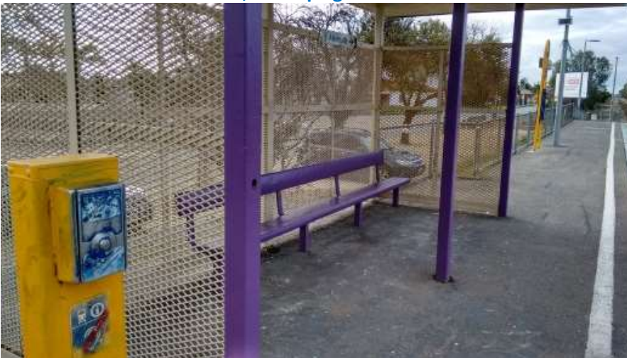
Photo 6. Steel mesh shelter , no help against a cold wind
